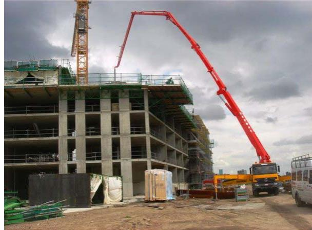
Figure 1b. Example of a commercial device to pour concrete in an on-service configuration.
