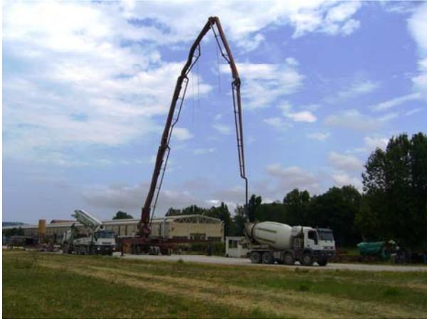
Figure 1a. Prototype of the five arm device produced in Romagna (the piping system to pour concrete can be easily seen).
