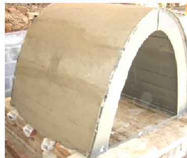
Figure 5. Replacement of refractory mass
