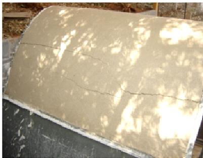
Figure 4. Fissure in the wall of the Oven 1
